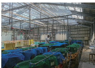
鴨池実験水槽 Kamoike land-based Aquaculture Facility
